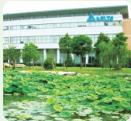
Plant Site Landscaping
