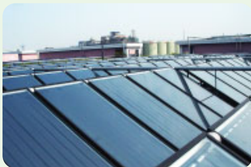
Solar Water Heating Systems
