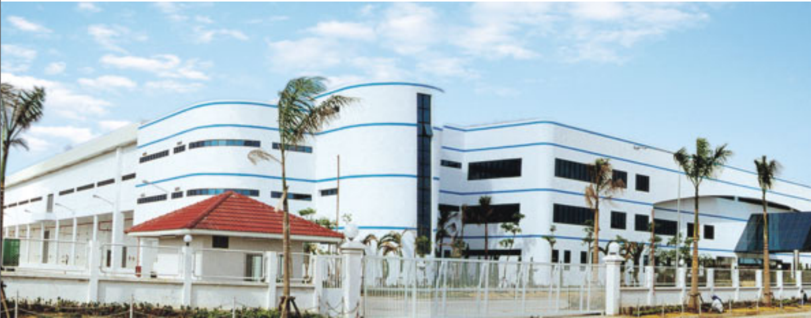
Power Supply Plant, Thailand
