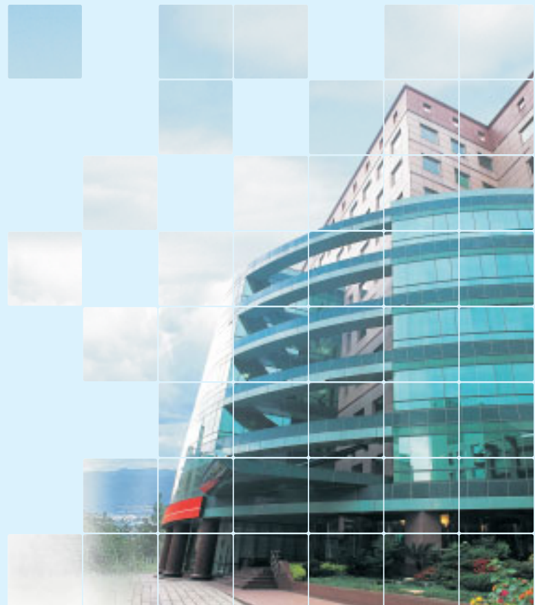
Delta Headquarters Entrance
